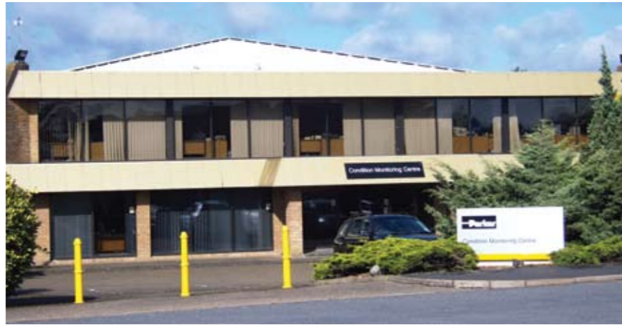
Condition Monitoring Business Unit, Thetford, UK
